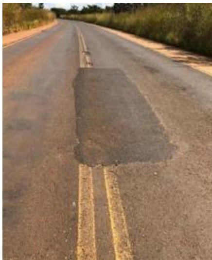
Figura 5 – Remendo [1]
